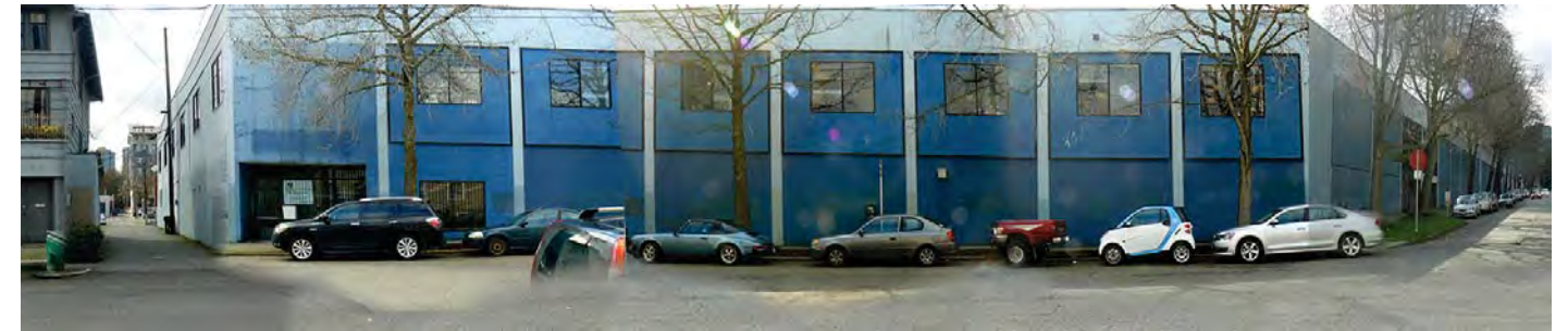
B View looking south from Harrison St.
