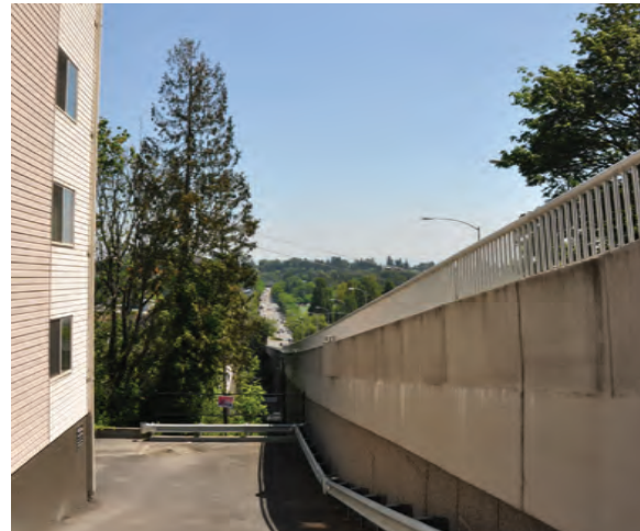
05. SITE, IN BACK LOOKING W | 2249 NE. 46TH ST.
