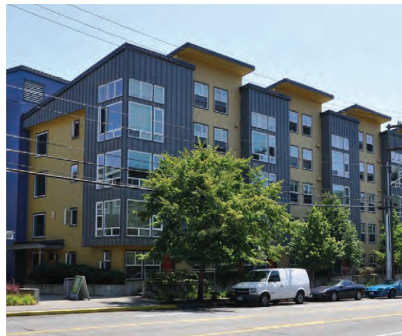
09. NORDHEIM COURT | 5000 25TH AVE. NE.
