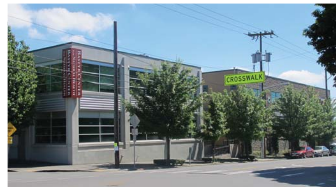
⑩ N 38TH & STONEWAY LOOKING SOUTHEAST
