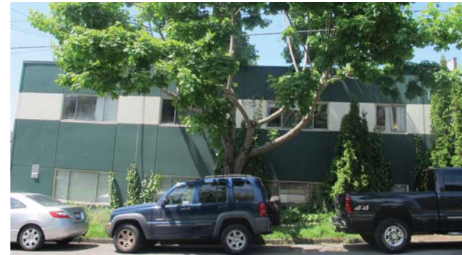
④ ADJACENT SITE TO SOUTH, LOOKING WEST
