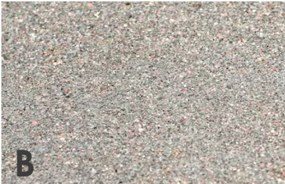
Concrete Paving (Exposed Aggregate Finish)
