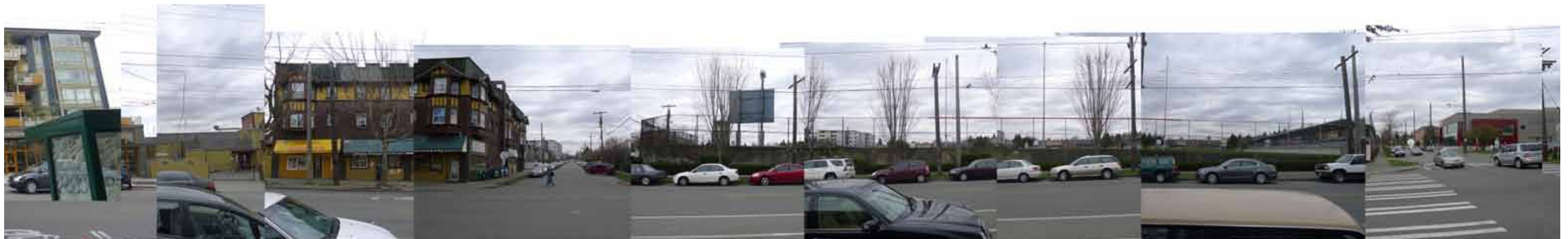
EAST JEFFERSON STREET LOOKING NORTH
