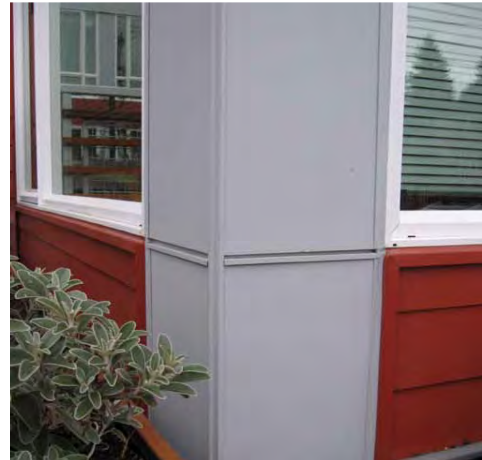
EXTERIOR PANEL JOINT & MIXED MATERIAL JOINT
