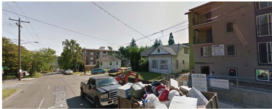
A VIEW FROM SITE WEST ACROSS 7TH AVE NE
