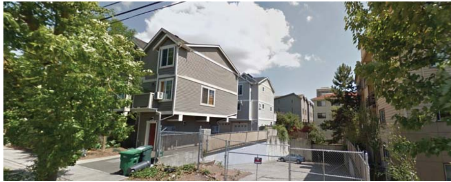
A VIEW EAST ACROSS 7TH AVE NE
