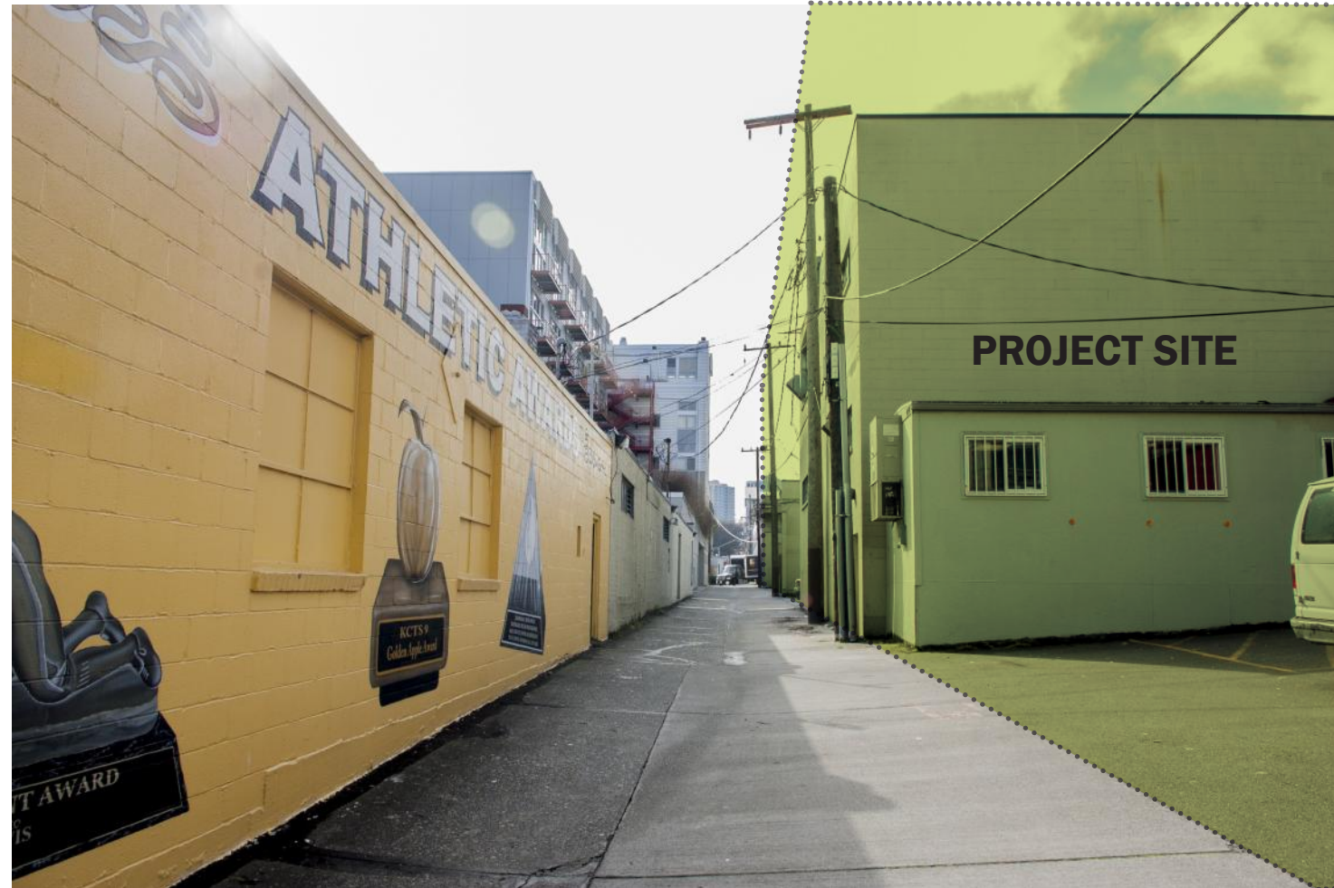
ALLEY - VIEW LOOKING SOUTH FROM REPUBLICAN STREET
