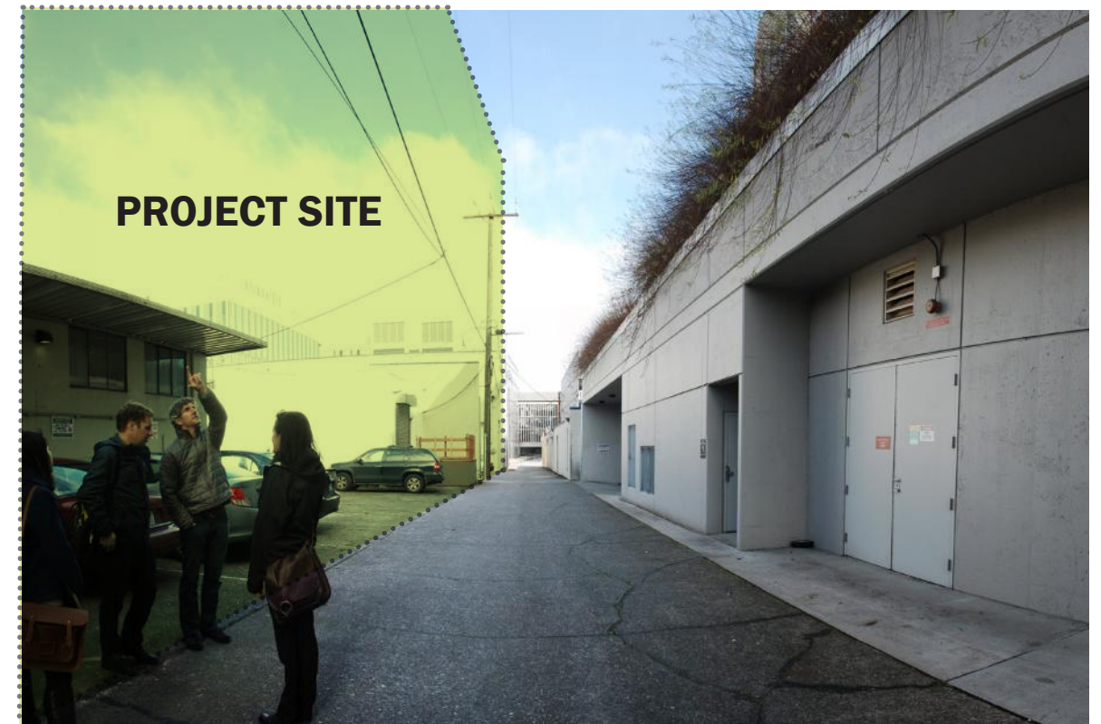
ALLEY - EXISTING CONDITION LOOKING NORTH FROM HARRISON STREET
