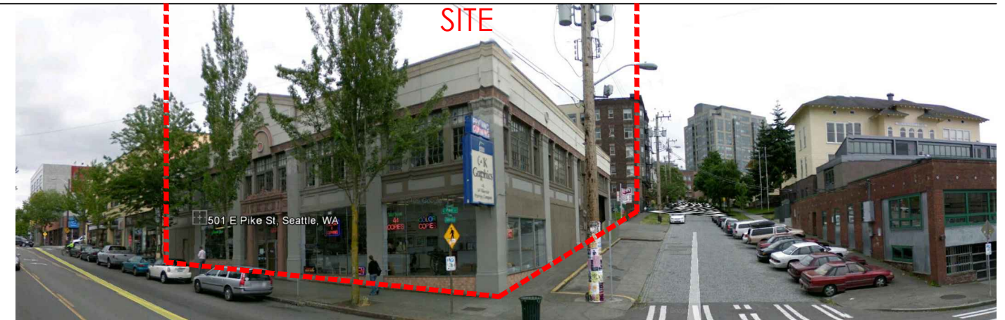
PROJECT SITE - CORNER OF EAST PIKE STREET & SUMMIT AVENUE
