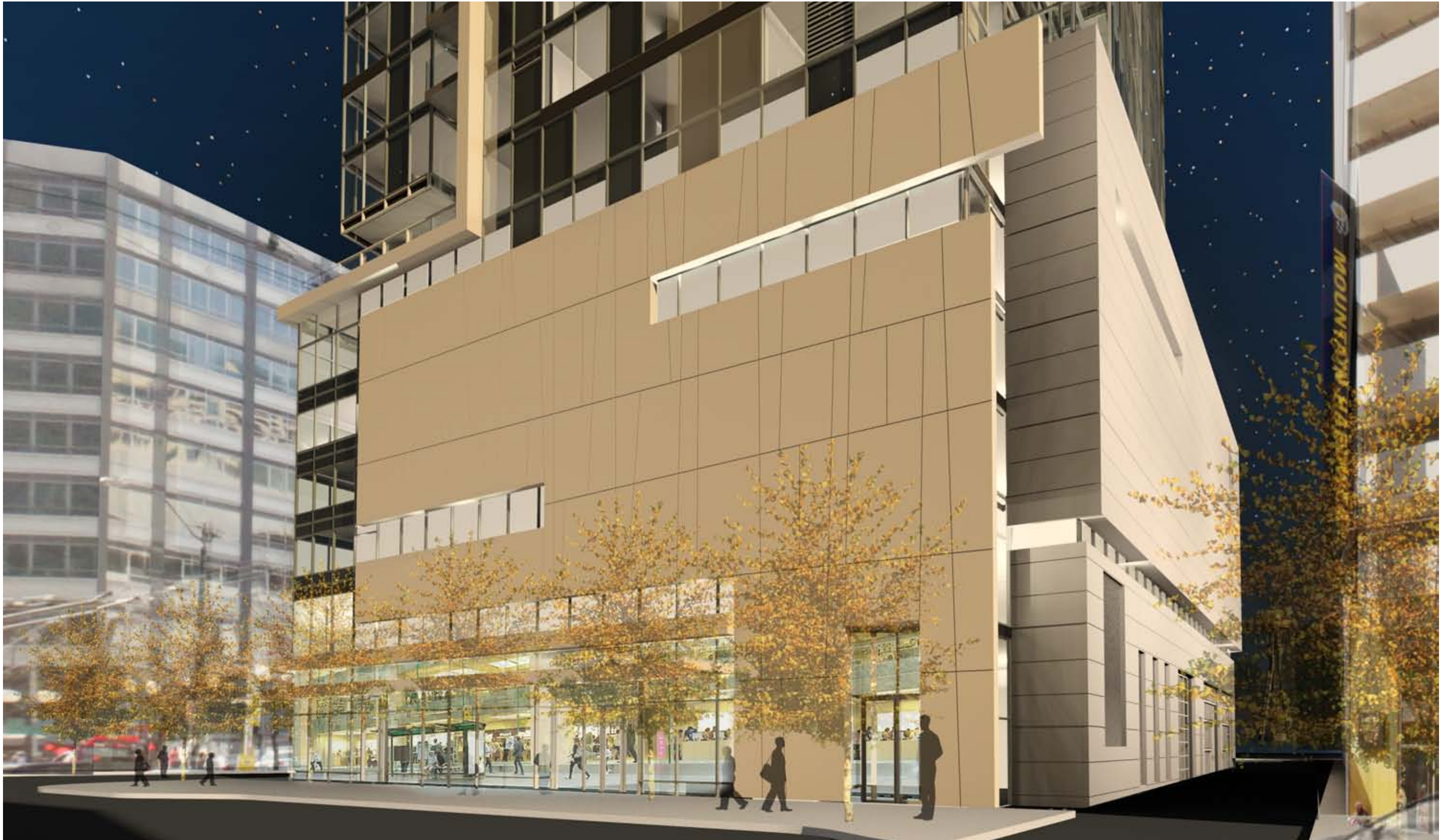
PODIUM VIEW AT NIGHT FROM SOUTHEAST
