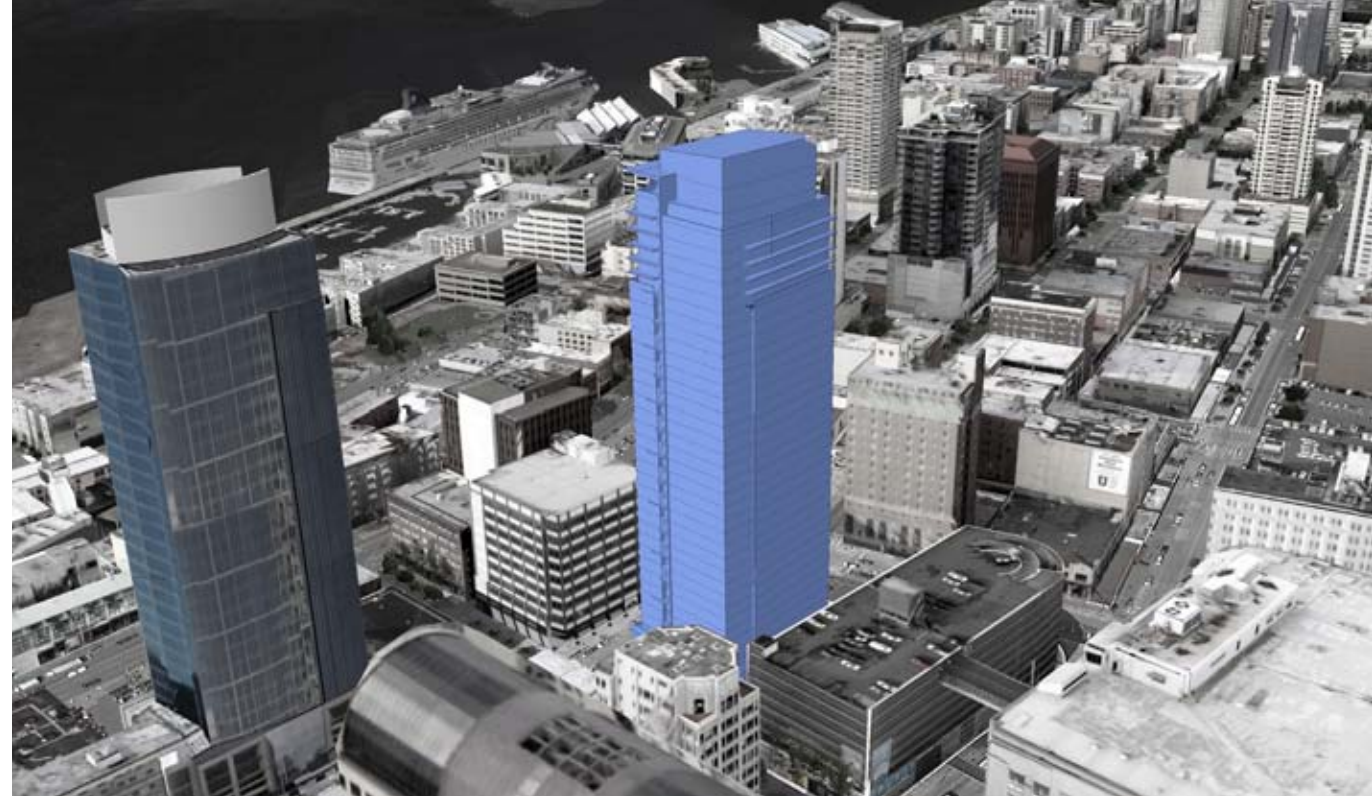
AERIAL VIEW FROM EAST
