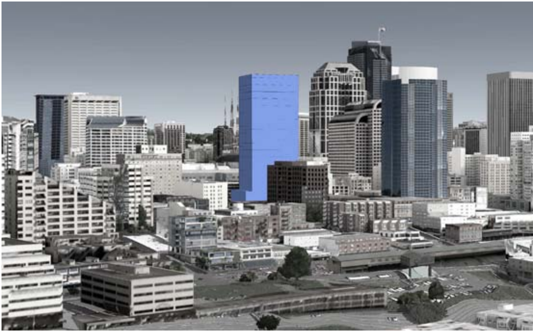
VIEW OF SITE FROM WEST
