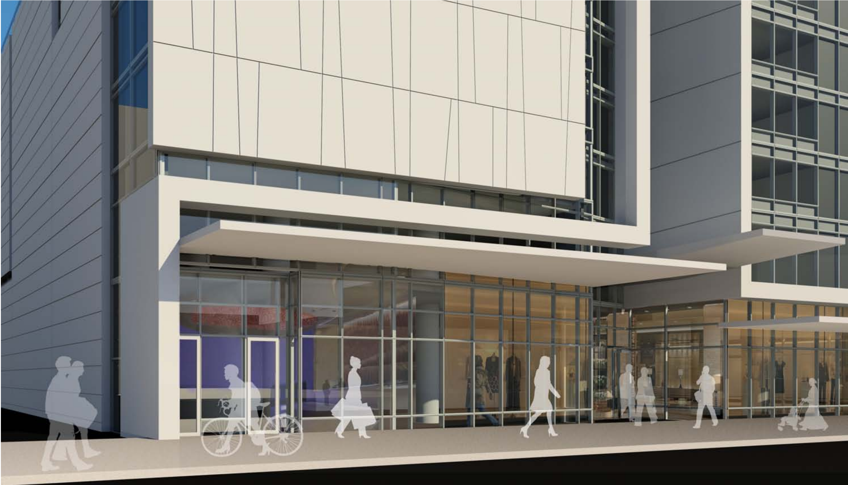
STREET LEVEL DETAIL AT CORNER OF NORTH FACADE AND SECOND AVENUE
