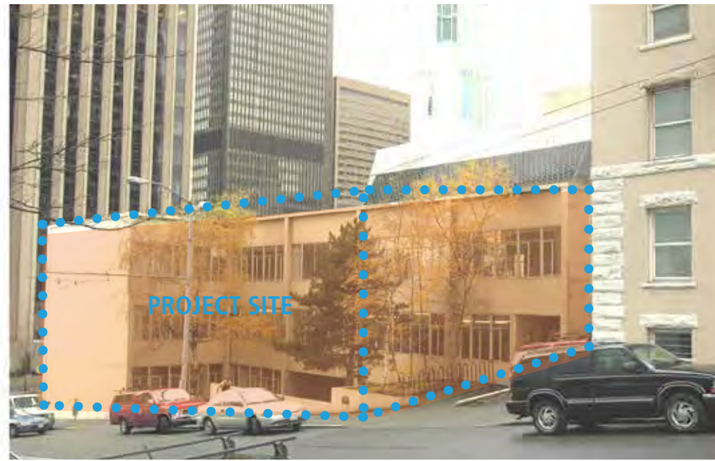
2 | View from Marion Street
