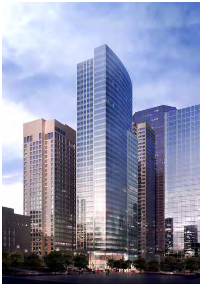
2008 VIEW OF 5TH AVE. AND MADISON ST CORNER
