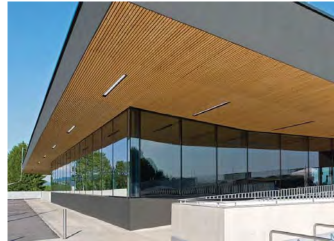
Lighting Concept at SE Corner Canopy
