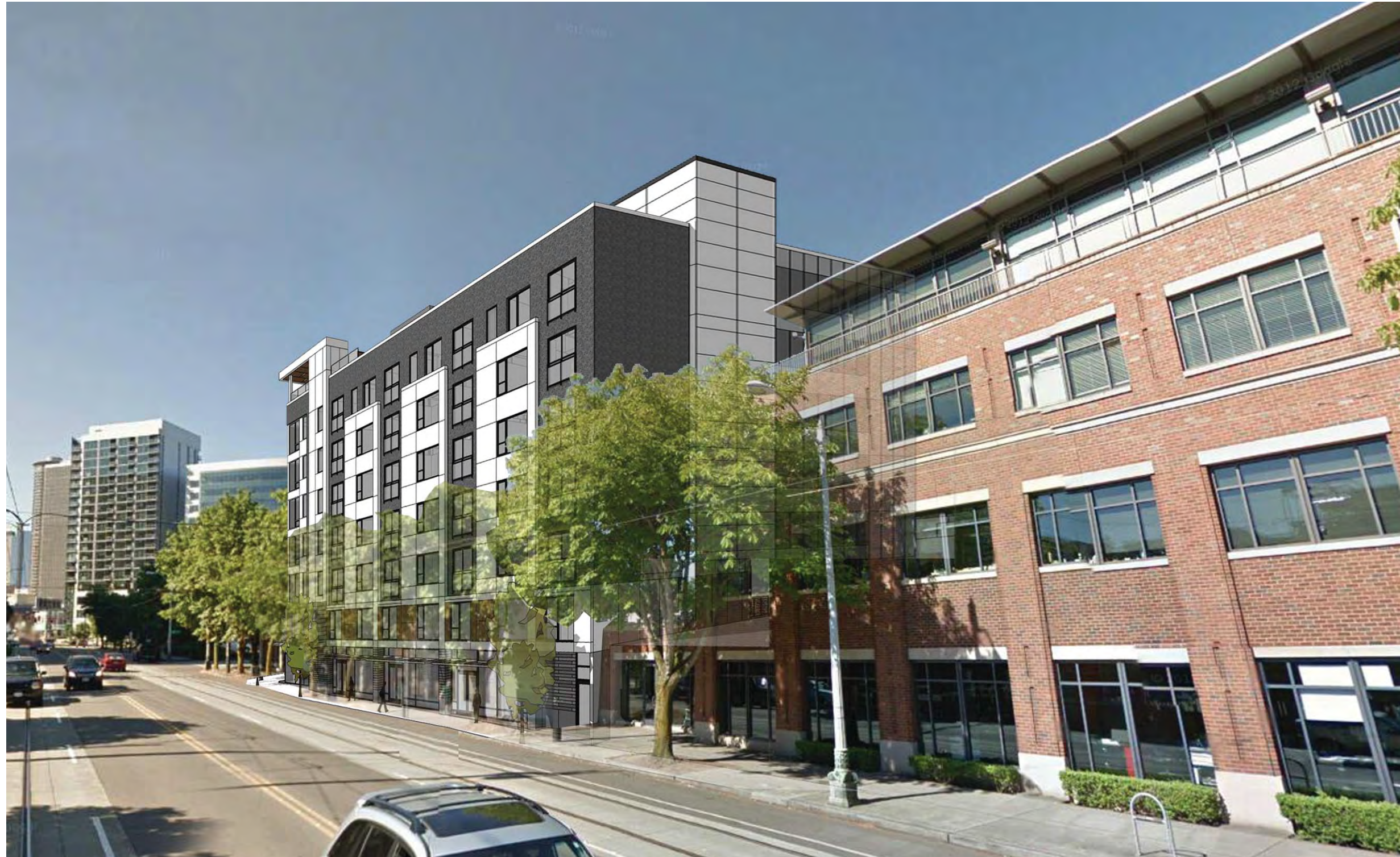
View of North Facade from Westlake
