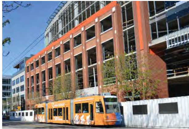
Vertical Bays Along Westlake / Brick
