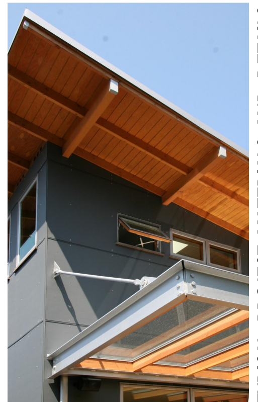
EXPOSED FRAMING ON ROOF OVERHANGS
