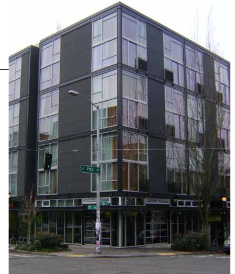
1 | corner expression & large amounts of glazing
