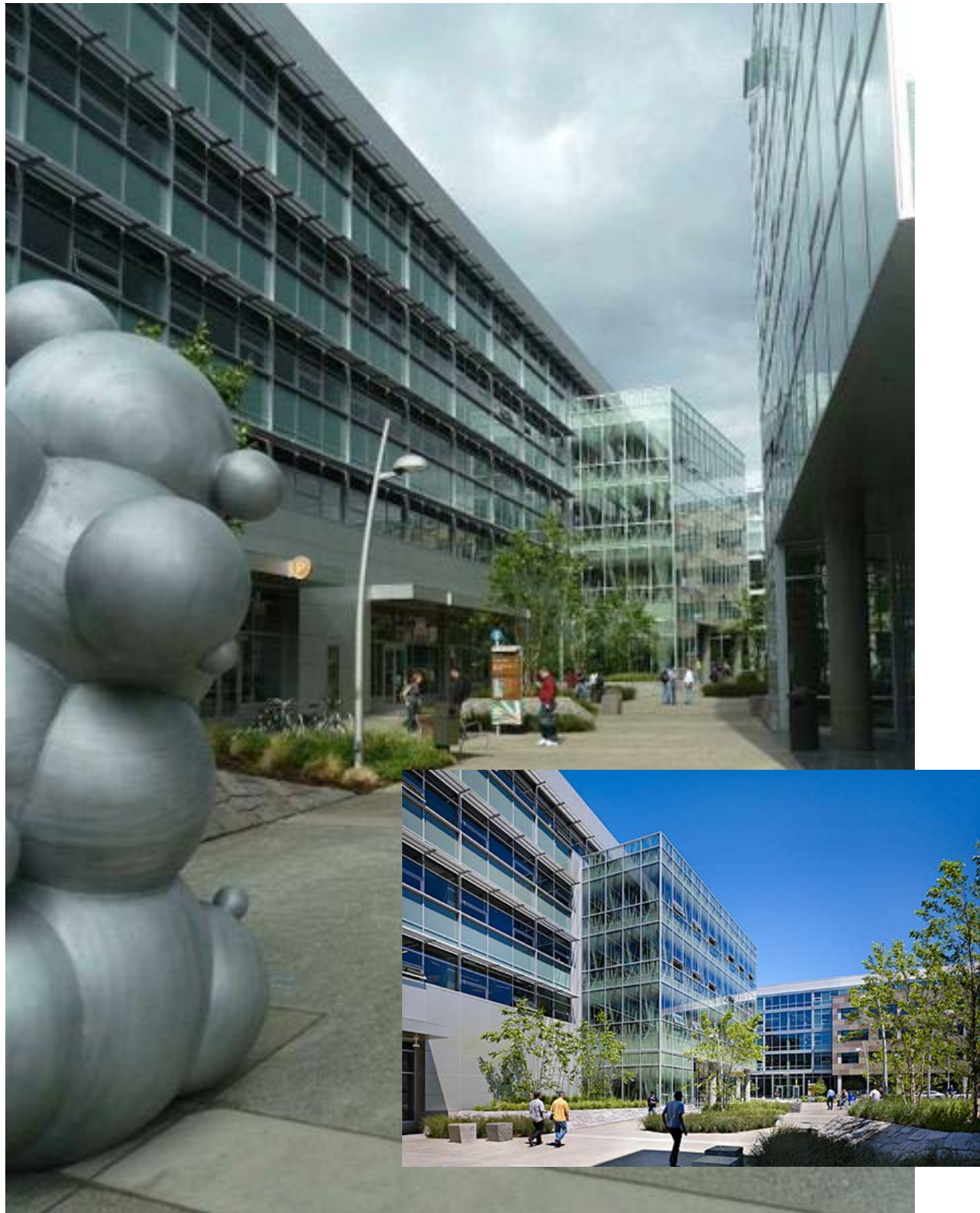
As part of the Amazon Campus, Phase III implements horizontal sunshades on the south facade, a unique grass inspired frit pattern on the glass, and public placement of sculptural art work.
