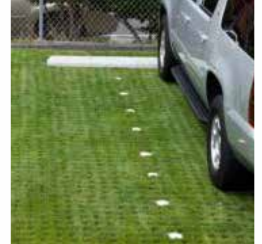
a paver of contrasting color or roadway dot may be used to define parking spaces. (image of plantable concrete systems from Soil Retention)
