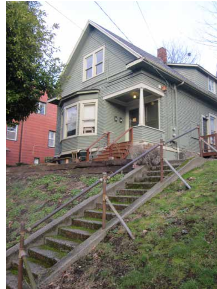
③ Existing structure on north side of lot
