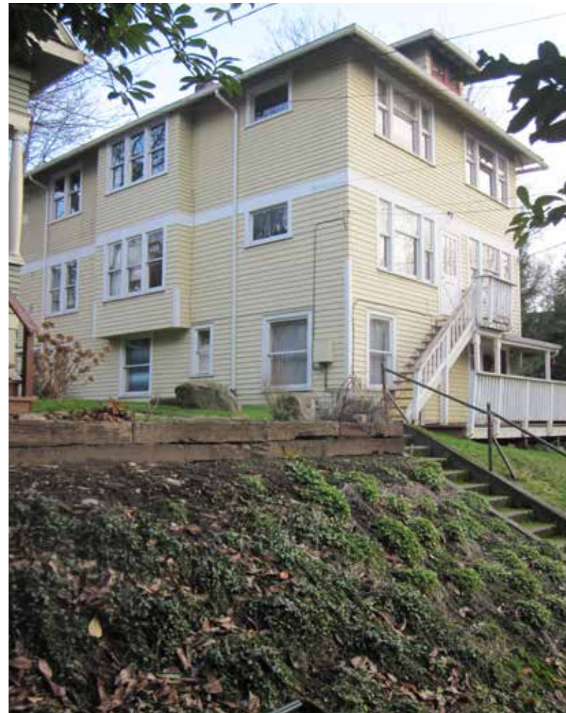
② Existing structure on south side of lot
