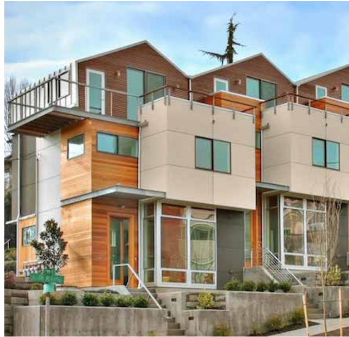
Planter walls of varying heights combine with front stoops provide a transition and buffer to the sidewalk.
