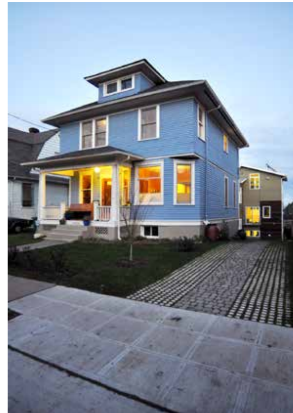
② 1504 19th Avenue Duplex behind SF House
