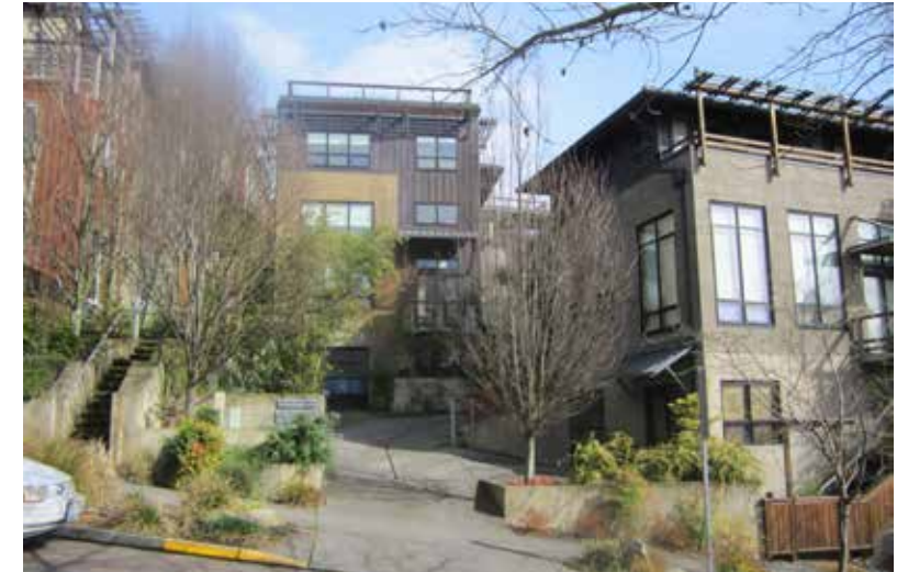
⑪ Multi-family building on Evanston Ave N
