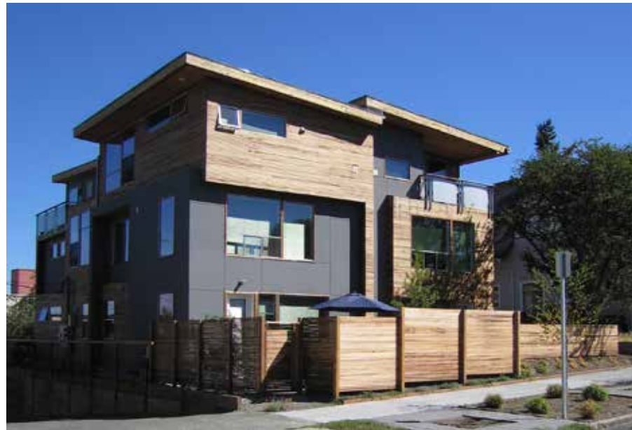
① 208 18th Ave. E. exterior view from street
