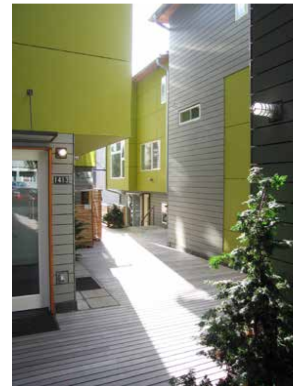
⑥ 1411 E. Fir St. interior boardwalk view
