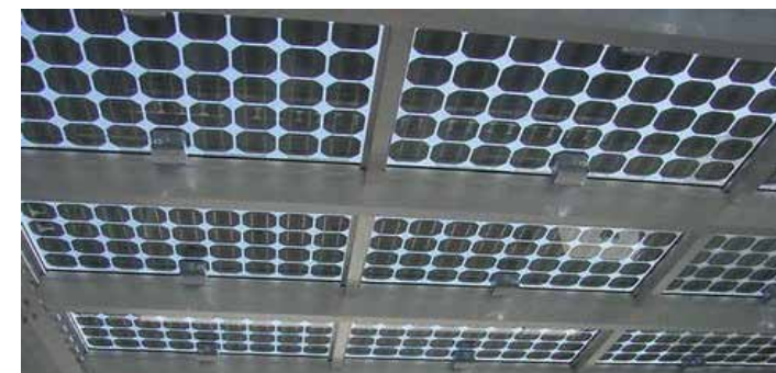
Example of horizontal sun shades with solar-panel
