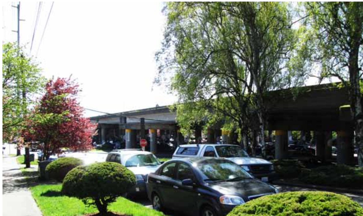
8TH AVE NE LOOKING SOUTH TOWARDS PARK AND RIDE
