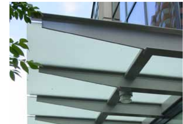
② Main entry canopy
