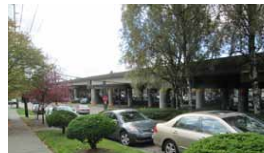
Photo of I-5 bridge immediately to the southwest of the project site.
