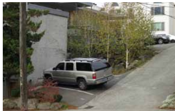
① BLANK WALL ON ADJACENT BLDG
