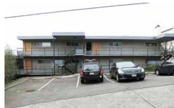
③ EXIT CORRIDOR ON ADJACENT BLDG
