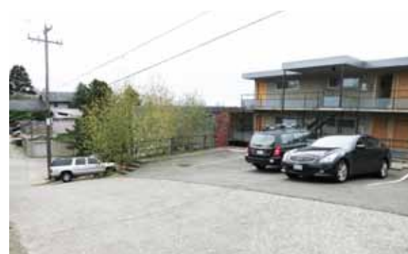
② ADJACENT BUILDING PARKING LOT
