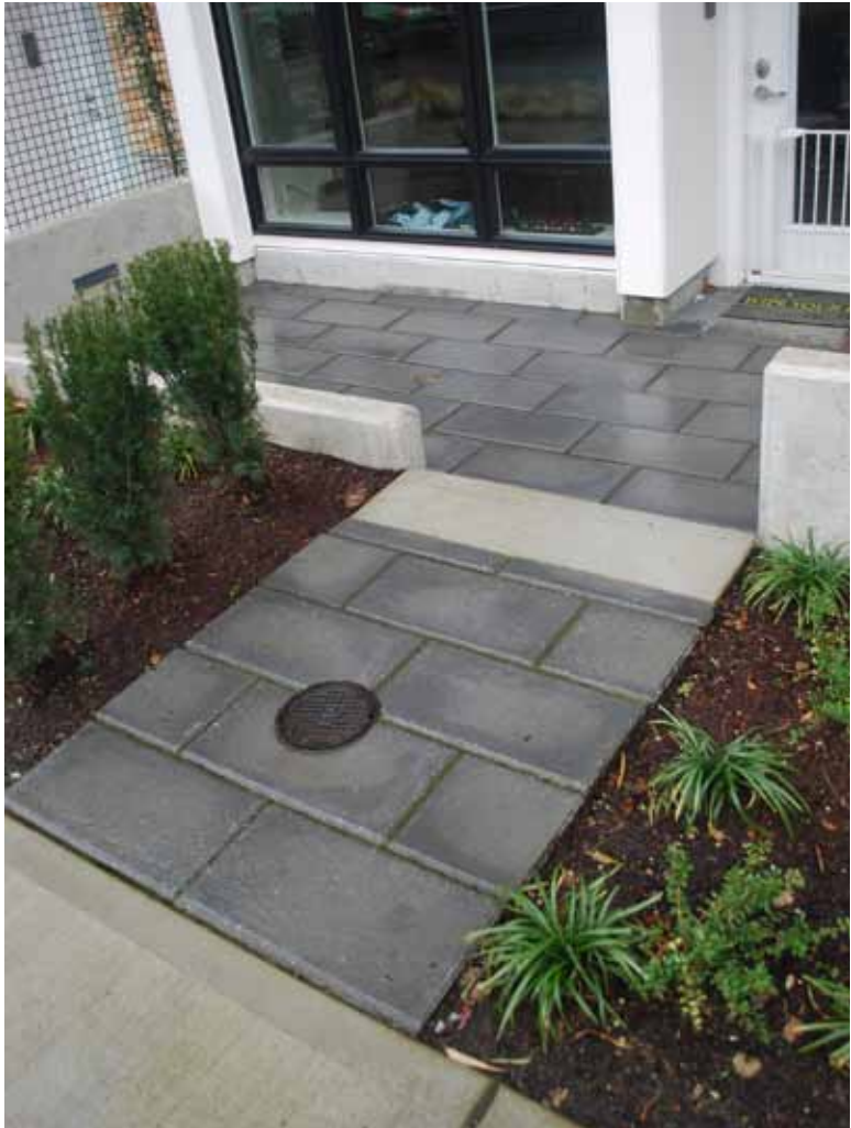
④ COMMERCIAL ENTRANCE - CONCRETE PAVERS
