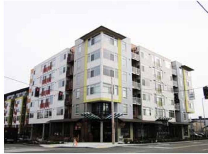
② LINK APARTMENTS
