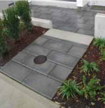
F CONCRETE PAVERS
