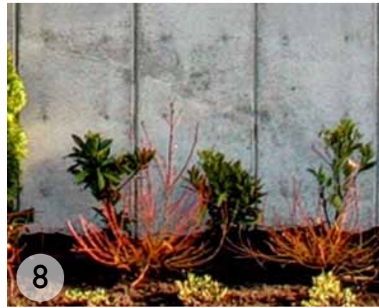
8 EXPOSED ARCHITECTURAL CONCRETE
