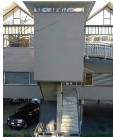
4 WCI Parking Stair
