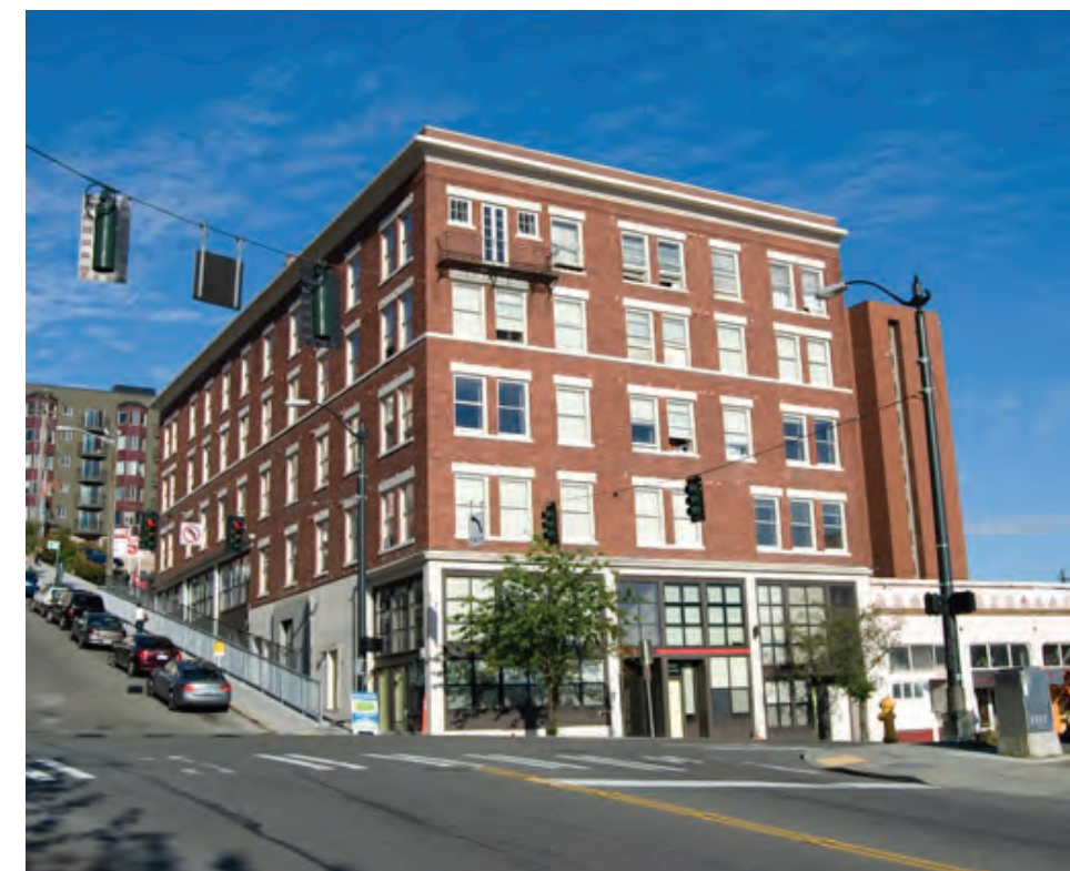
Ascona Apartments, Seattle: major rehabilitation of existing brick apartment building. Developer: Daly Partners
