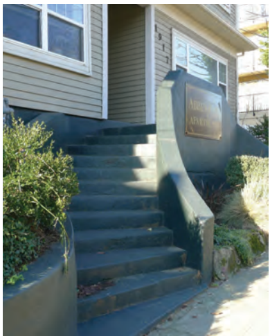
5 Abbey Park Apts Entry Stairs
