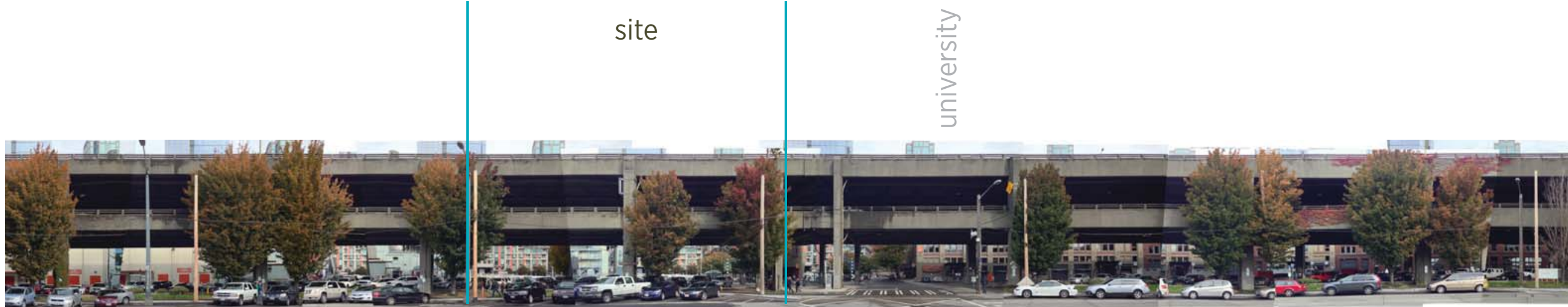
looking east: to be replaced with treed boulevard
