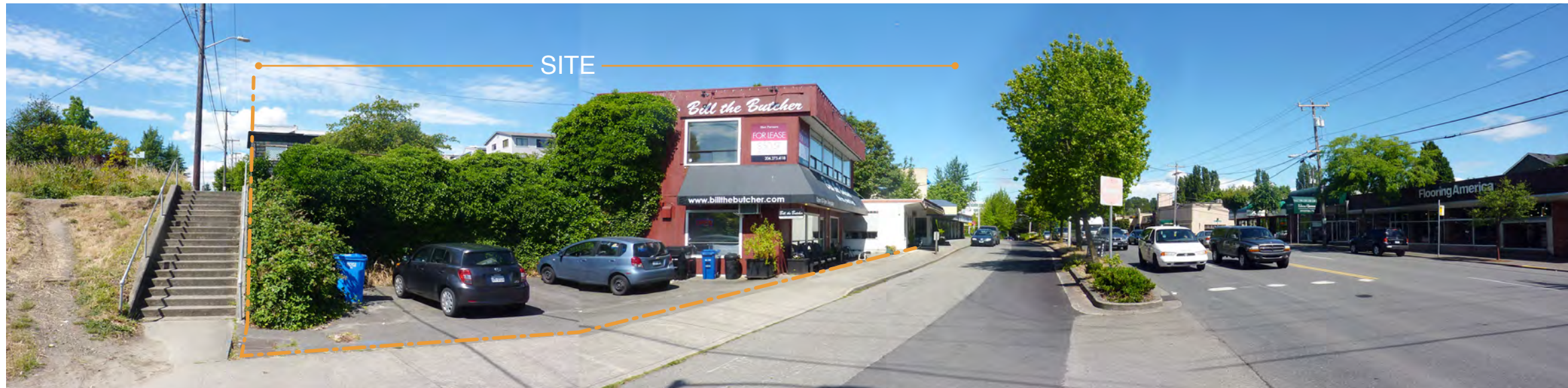
1. Existing condition from 45th Street and 36th Ave NE
