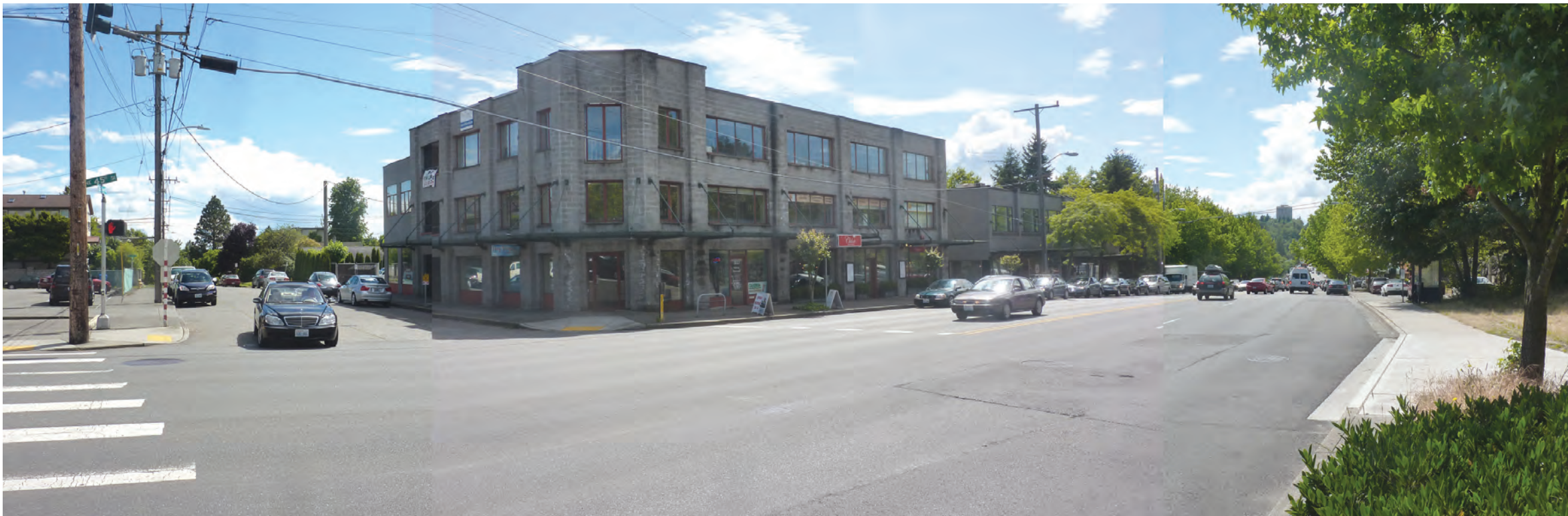
Looking Southwest at NE 45th & 36th Ave NE
