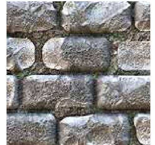
cobblestone paver at garage entry
