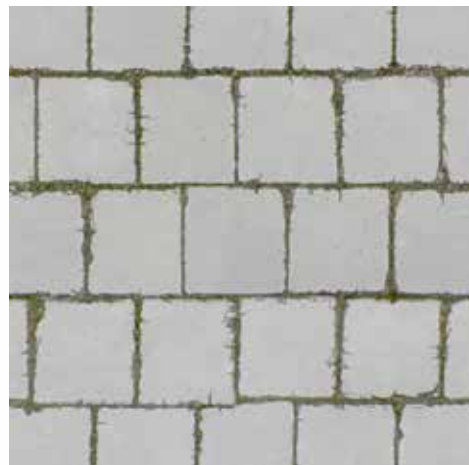
pavers at courtyard
