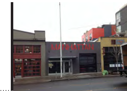
Garlick Building / Manhattan year | 1920, renovated 2005 restaurant
