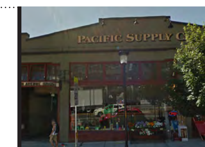
Pacific Supply Co. Building year | 1920, renovated 2002-2004 retail/industrial
