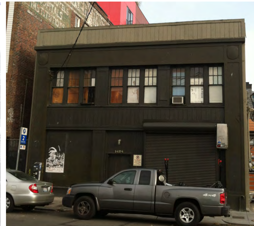
The building in its current condition has been overlaid with T-111 siding at the parapet and spandrel.
