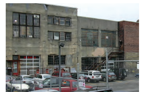
6) 11th Avenue east side looking at rear facades of buildings facing 12th Avenue
