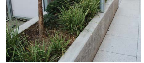
CIP Concrete Seatwall
