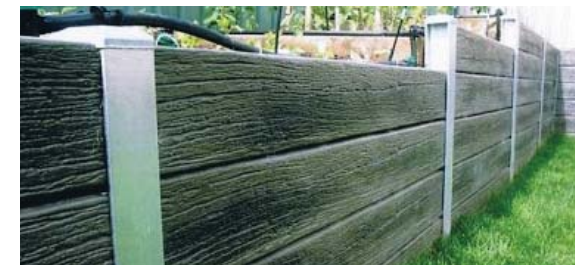
Timber/Pile Retaining Wall
