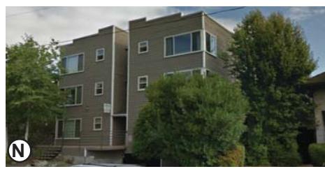
The Wallingford Apartments Residential
