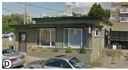
1902 N 34th St. Office
