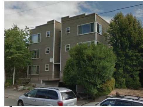
The Wallingford Apartments
