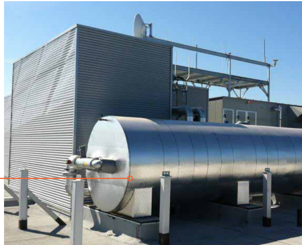
PHASE CHANGE THERMAL STORAGE AT FEDERAL CENTER SOUTH
