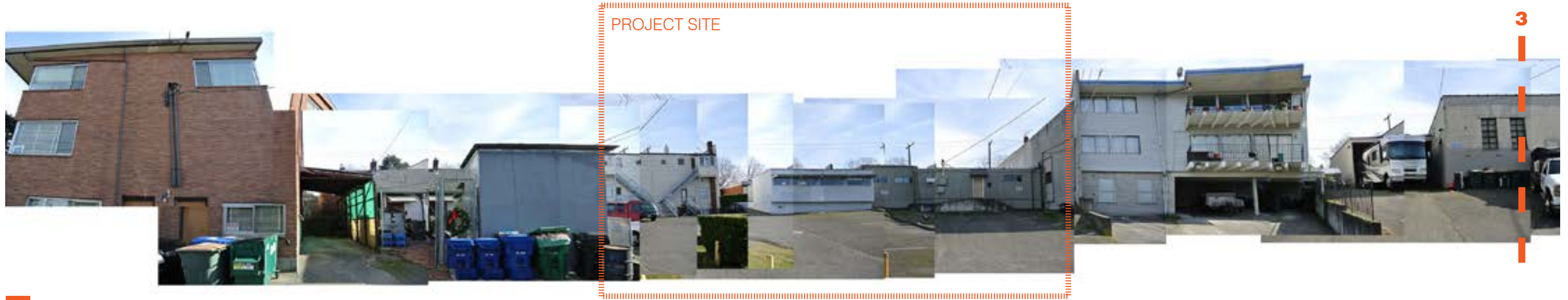
3 ALLEY LOOKING EAST
