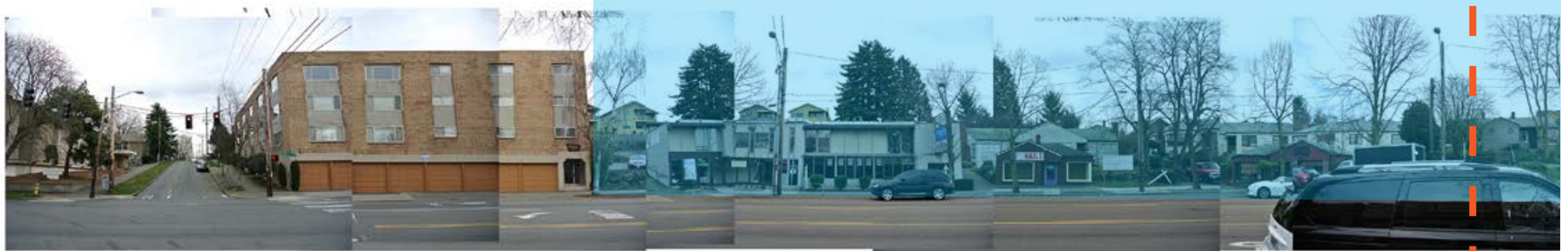
2 CALIFORNIA AVENUE S.W. LOOKING EAST
