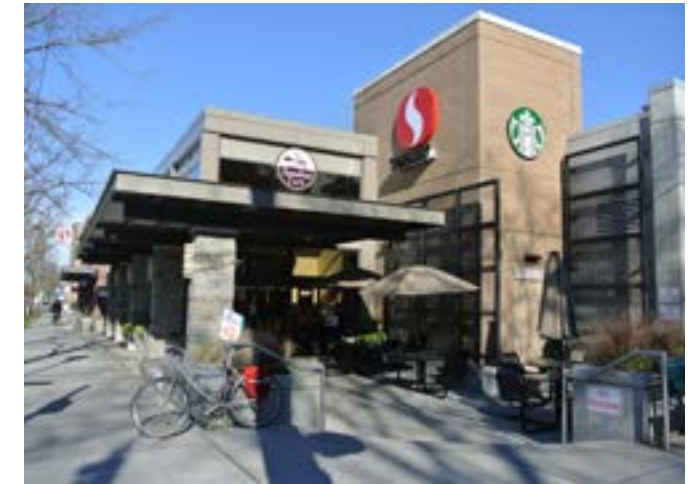
13 ELEMENT 42 / SAFEWAY: MIXED-USE PROJECT
