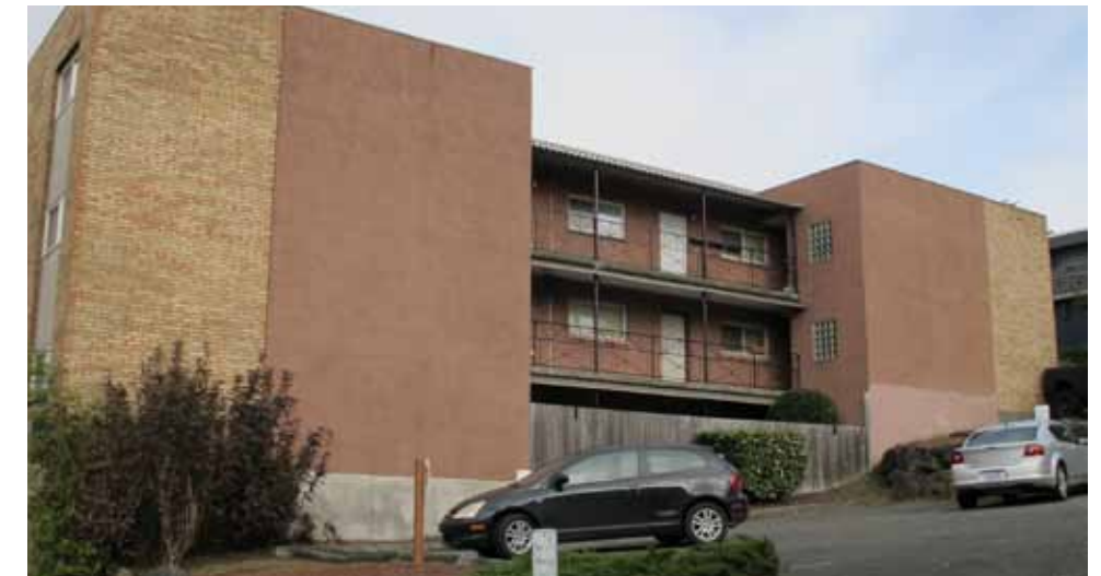
④ ADJACENT MULTI-FAMILY STRUCTURE AT NORTH PROPERTY LINE
