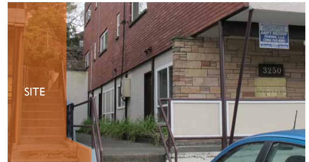
⑤ SOUTH PROPERTY LINE SHOWING CHANGES IN GRADE
