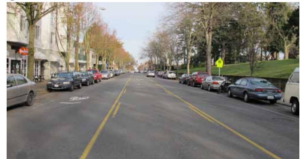
⑪ LOOKING NORTH ALONG CALIFORNIA AVE. SW
