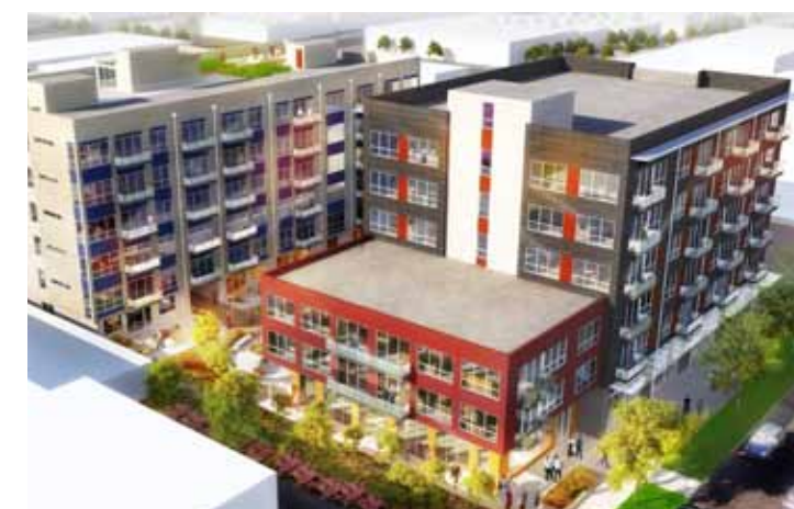
BROADSTONE KOI - LEED-NC CERTIFIED TARGET
