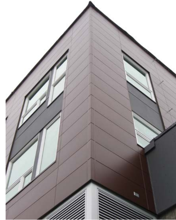
Fiber Cement Panel with Concealed Fasteners
