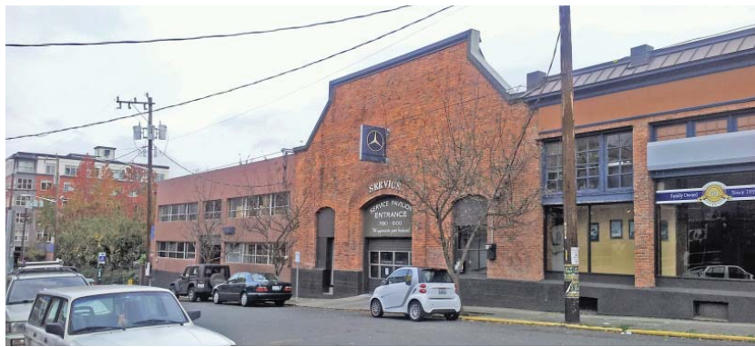
Conserve historic facade of Bldg #3
