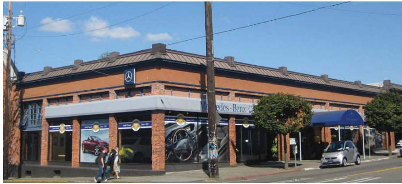
Conserve historic facades of Bldg #1
