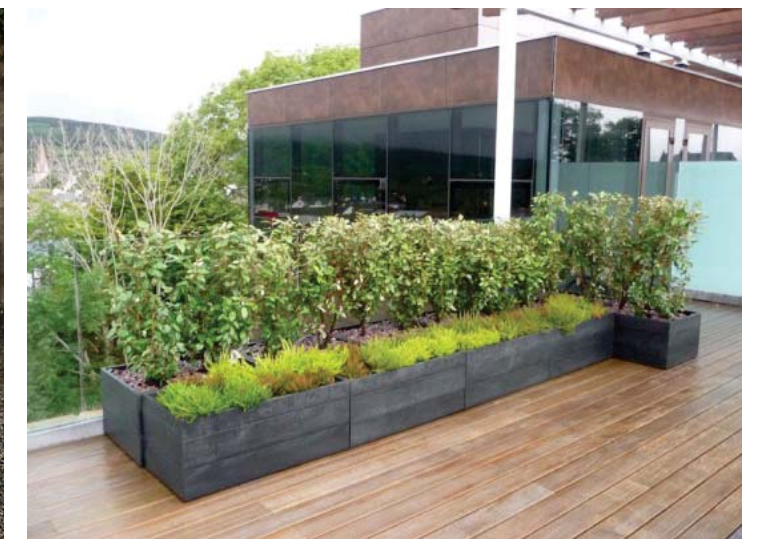
WOOD DECK & PLANTERS
