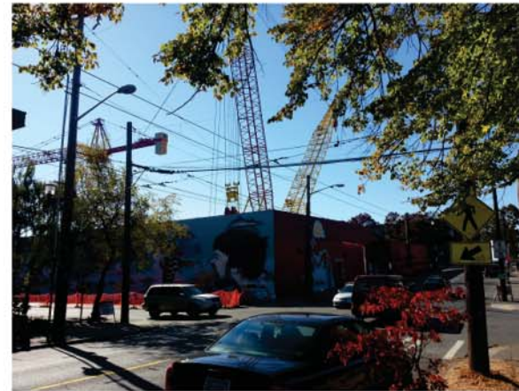
5. NEW LIGHT RAIL STATION SITE
