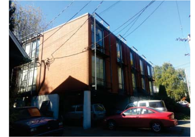
11. E. JOHN ST. LOOKING SW
