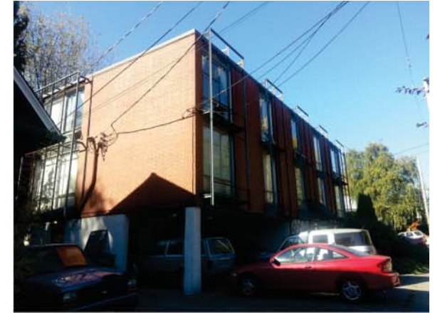
11. E. JOHN ST. LOOKING SW
