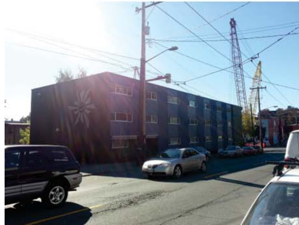
1. E. JOHN ST. LOOKING SW
