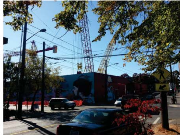
5. NEW LIGHT RAIL STATION SITE
