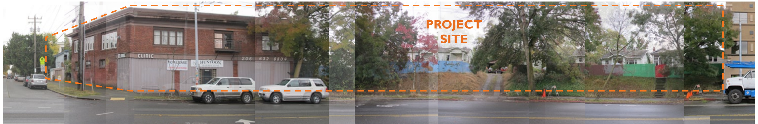
LOOKING SOUTH AT N 45TH STREET AND INTERLAKE AVENUE
