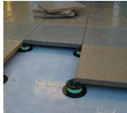
E ARCHITECTURAL SLAB PAVING 24"x24" (TYP.)
