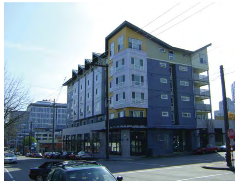
BUILDING JUST EAST OF OUR PROJECT DID NOT SET BACK ALONG THOMAS ST
