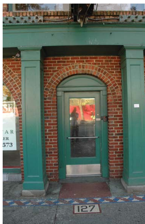
2. VIEW LOOKING WEST (EXISTING COMMERCIAL ENTRANCE)
