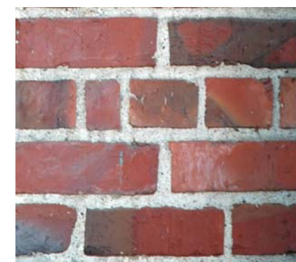
5 Existing Brick, East Wall
