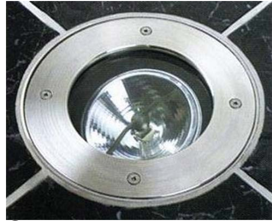
2 ARCHITECTURAL UPLIGHT - GRADE LEVEL COLUMNS AND SOUTH STAIR TOWER
