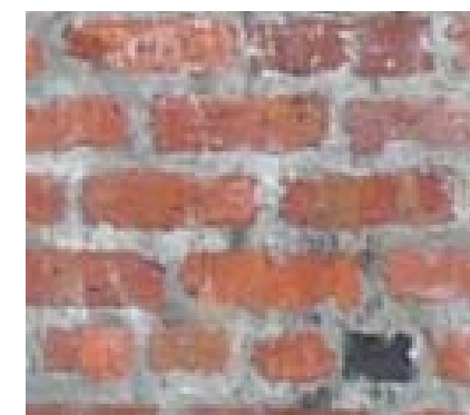
6 Existing Brick North, South & West Walls
