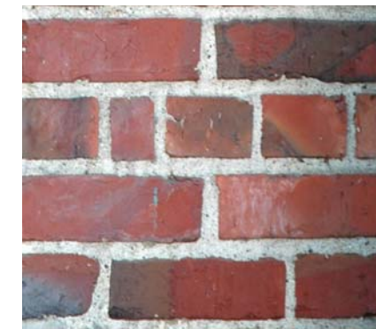
5 Existing Brick, East Wall
