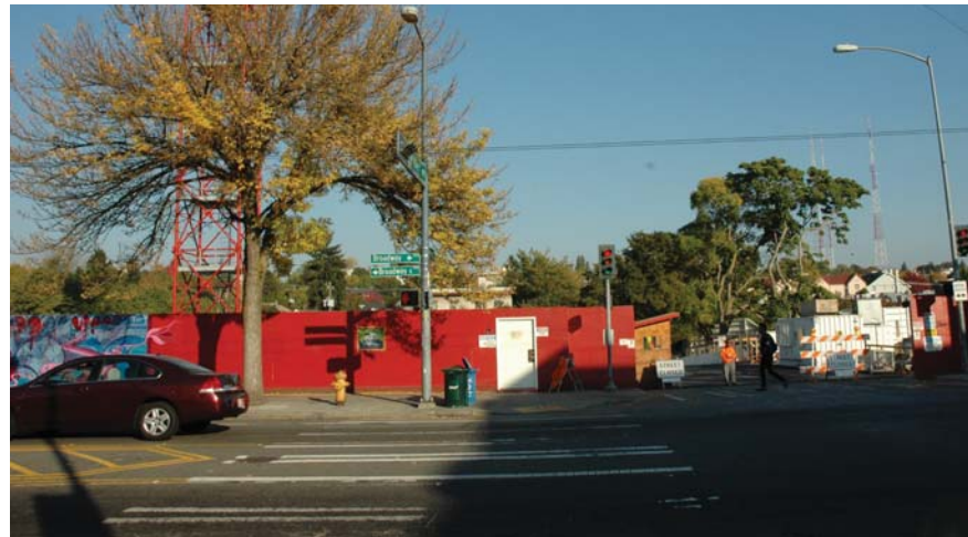
4. VIEW LOOKING EAST (FUTURE LIGHT RAIL STATION)
