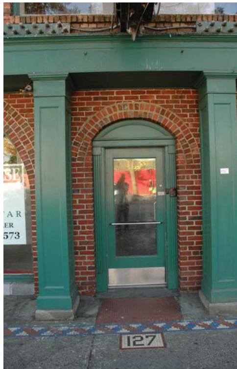
2. VIEW LOOKING WEST (EXISTING COMMERCIAL ENTRANCE)
