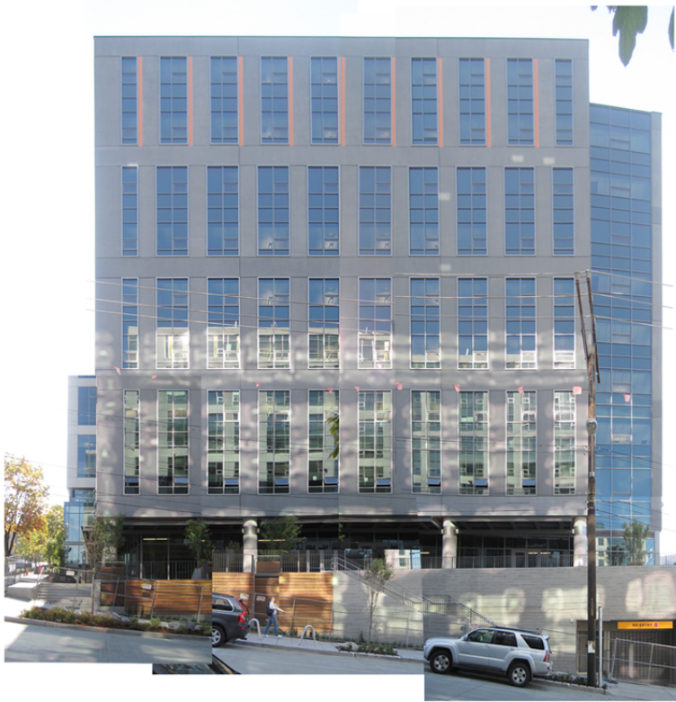
3. EXISTING STREETScape ALONG THOMAS STREET LOOKING SOUTH
