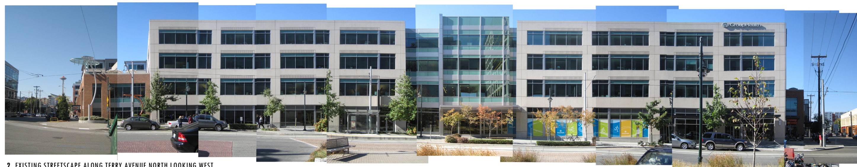
2. EXISTING STREETScape ALONG TERRY AVENUE NORTH LOOKING WEST
