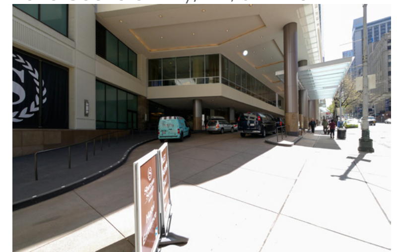
Porte Cochere, 6th Ave
