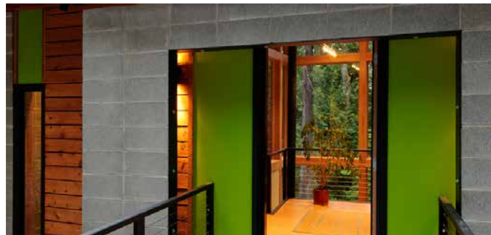
CONCRETE BLOCKS AND COLORFUL ENTRY
