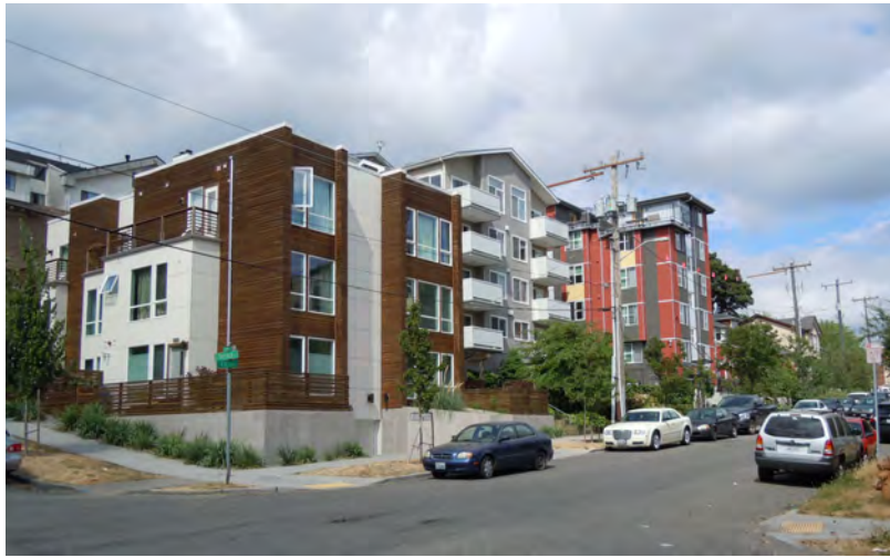
① Apartments on 11th Ave.
