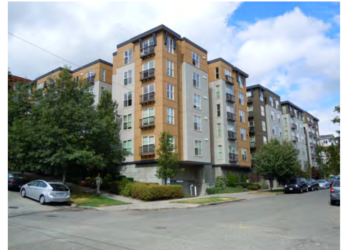
⑥ Apartment Building- 1011 E. Terrace St.
