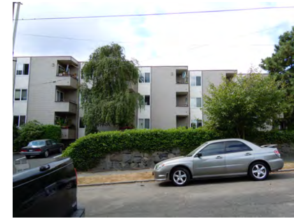
⑤ Alder House Apartments view from site
