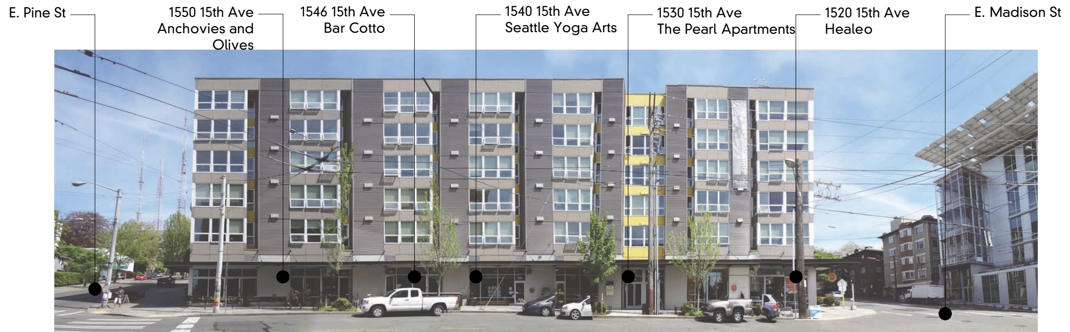
15th Avenue - East Side of Street
