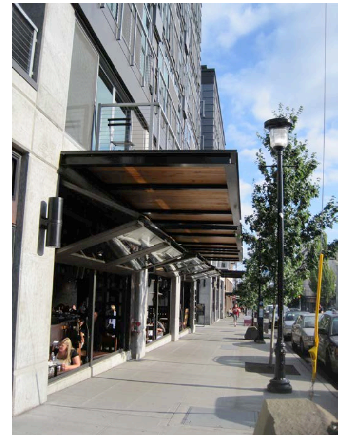
Steel Framed Awning with Cardecking Infill
