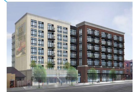
REO Flats - Under Construction
