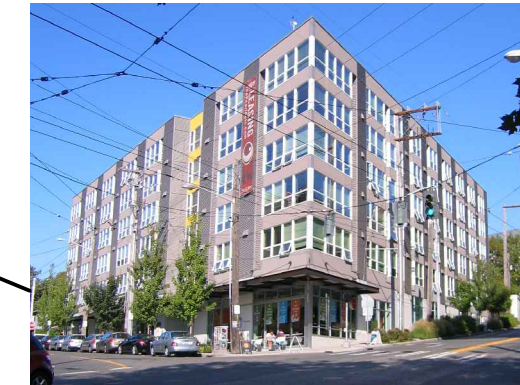
E MADISON LOOKING NE -MIXED USE, RETAIL ON 15TH METAL & CEMENTATIOUS SID'G
