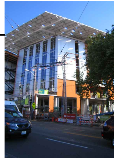
BULLITT FOUNDATION "LIVING BLDG" (UNDER CONSTRUCTION)
