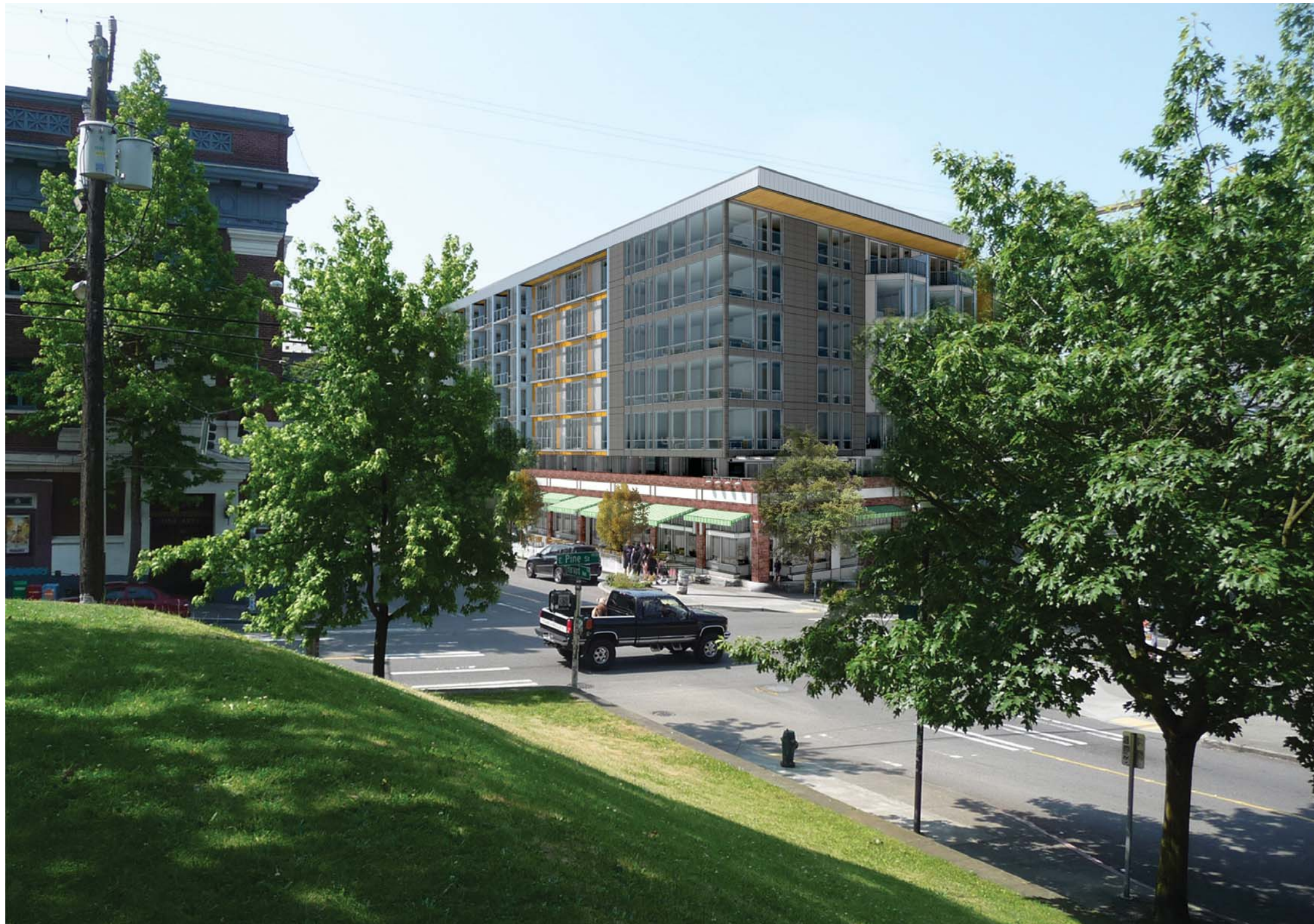
VIEW LOOKING SOUTHWEST FROM COMMUNITY COLLEGE
