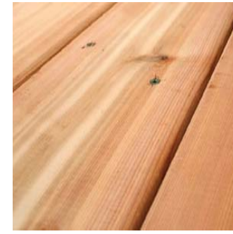
6 WOOD SOFFIT: CEDAR PLANKS
