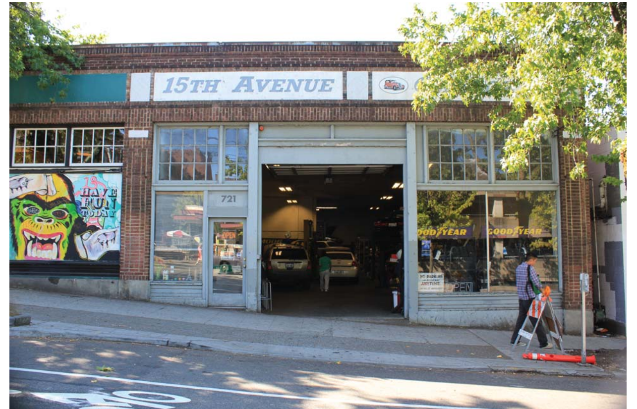
1. VIEW LOOKING SOUTH (15TH AVENUE GARAGE)
