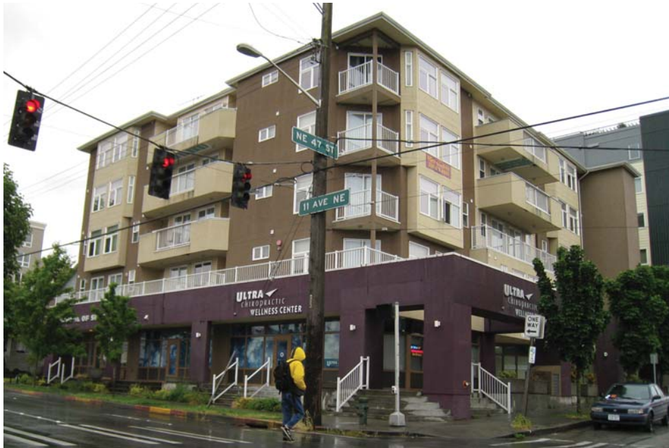
Sunrise Cascade Apartments 1100 NE 47th Street
