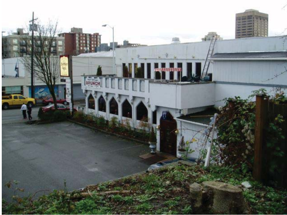
View of site from the west
