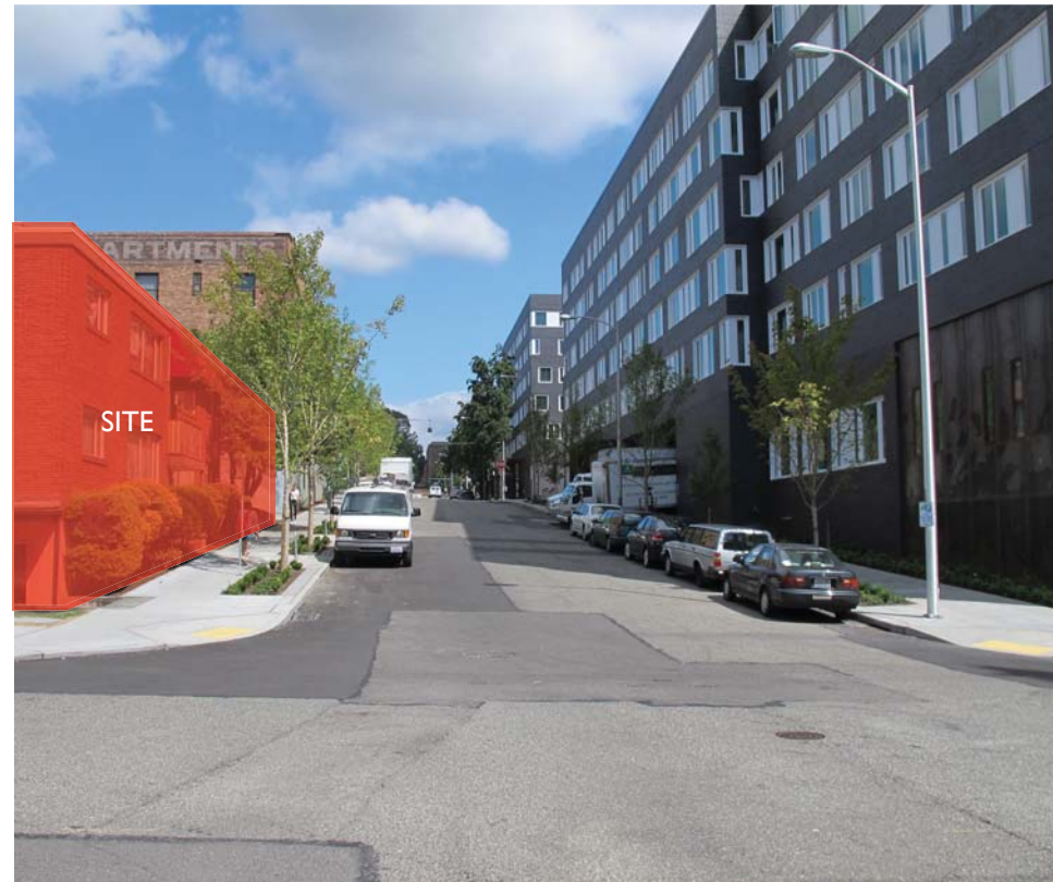
⑧ LOOKING EAST ALONG NE 41ST STREET
