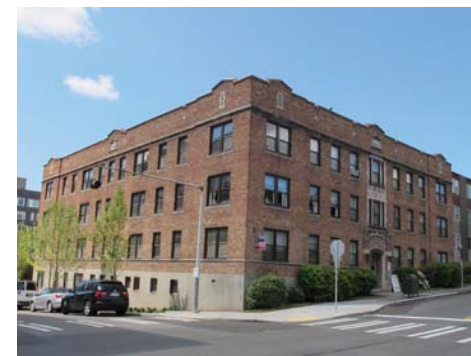
⑦ THE LEVERE APARTMENTS
