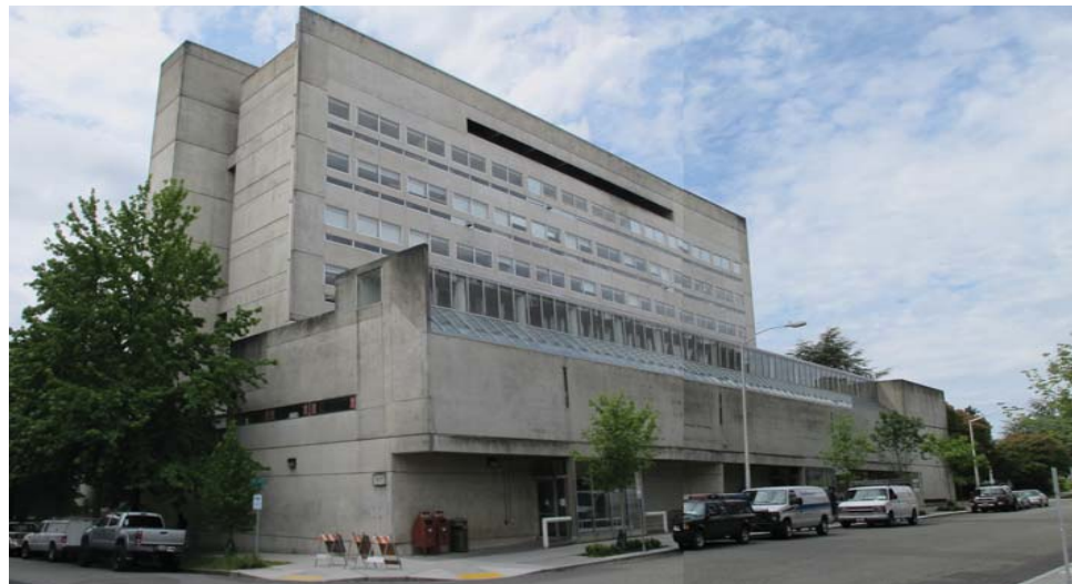
⑥ CONDON HALL FROM PROJECT SITE
