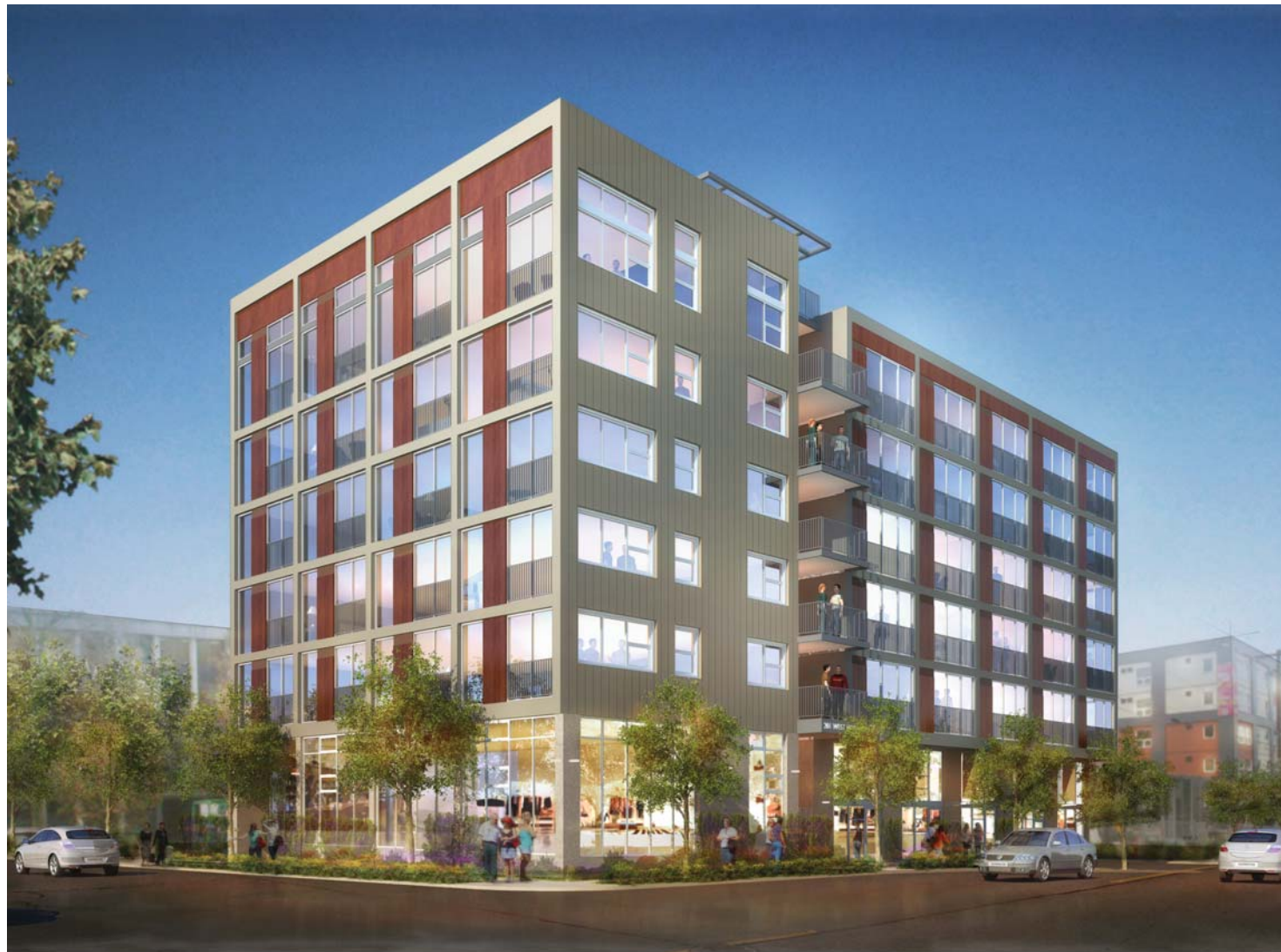
H2O APARTMENTS - LEED H MIDRISE PILOT GOLD TARGET
