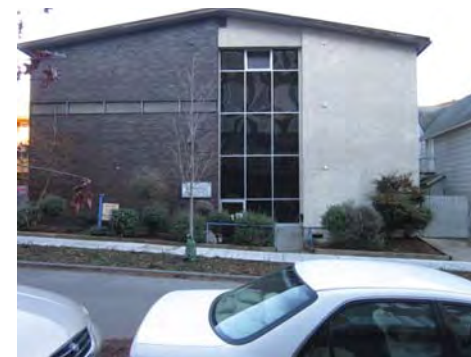
④ DEL CAPRI APARTMENTS
