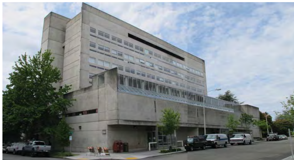
⑥ CONDON HALL FROM PROJECT SITE
